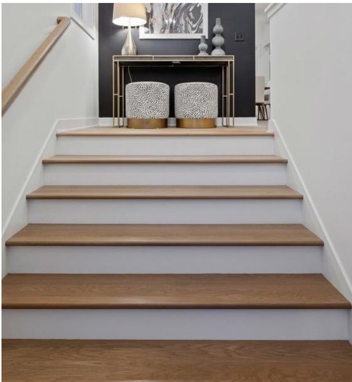
STAIRS: PAINTED RISERS, WOOD STAIRS & RAILING TO MATCH WOOD OR WOOD TILE FLOOR RAILING: SQUARE PROFILE STAINED TO MATCH
