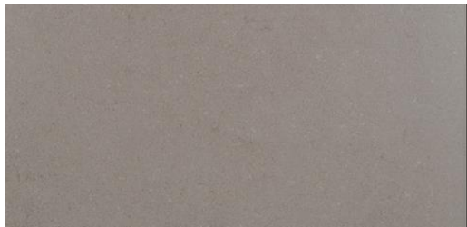
BATH 2 FLOOR: MSI DIMENSIONS GRIS 12"X24", INSTALLED STRAIGHT STACK GROUT #107 IRON
